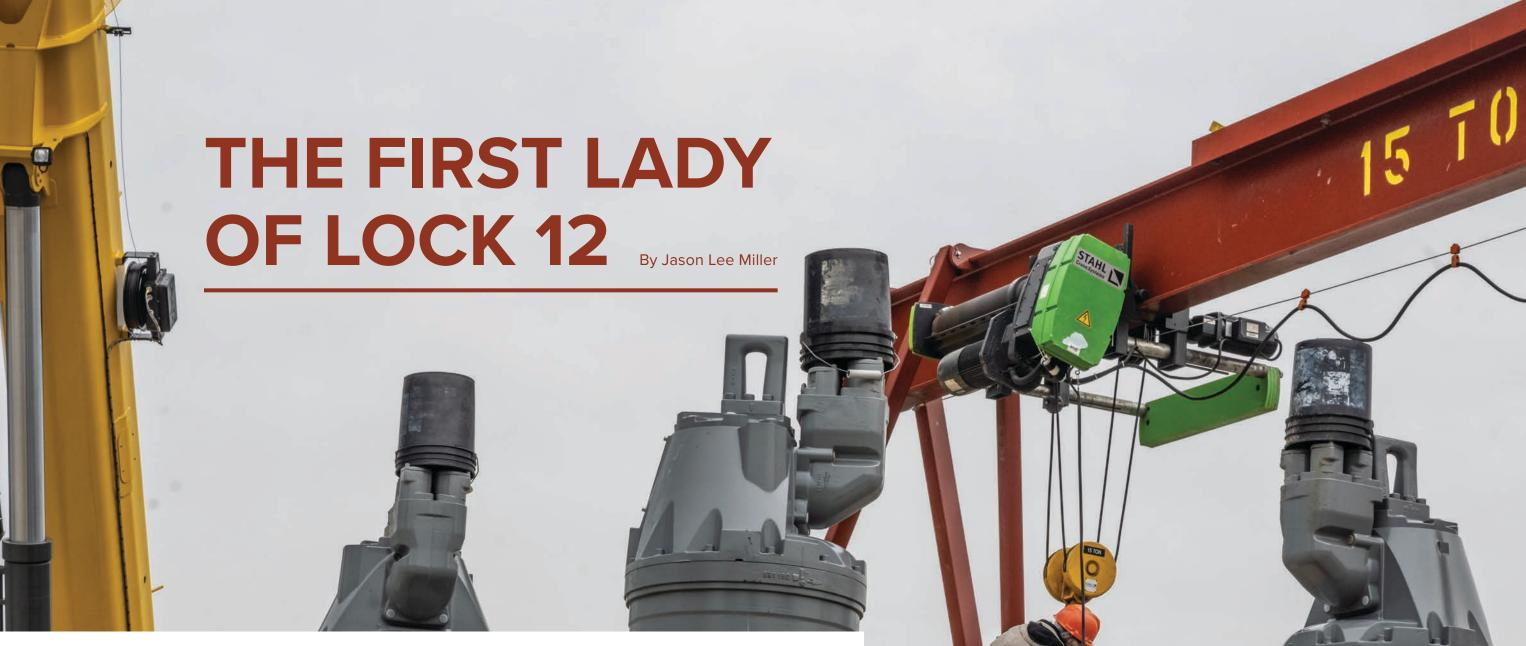
Iturbine generators are converting a million gallons of water per minute into clean electricity. The 13-foot tall, 23,000-pound turbine generators represent just some of the marvelous technology The grand design being used at the Matilda Hamilton Fee Hydroelectric Station, Kentucky in 94 years.
