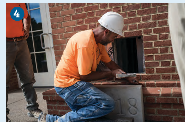
Masons came to the rescue, removing a course of brick at the lower edge of the opening.
