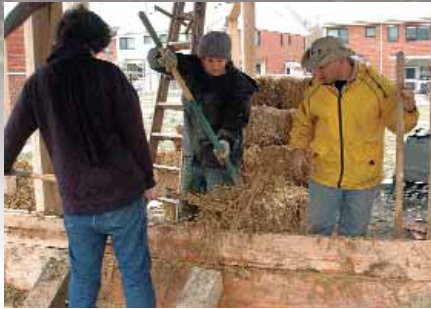
Straw bale construction of the Ecovillage solar shed
