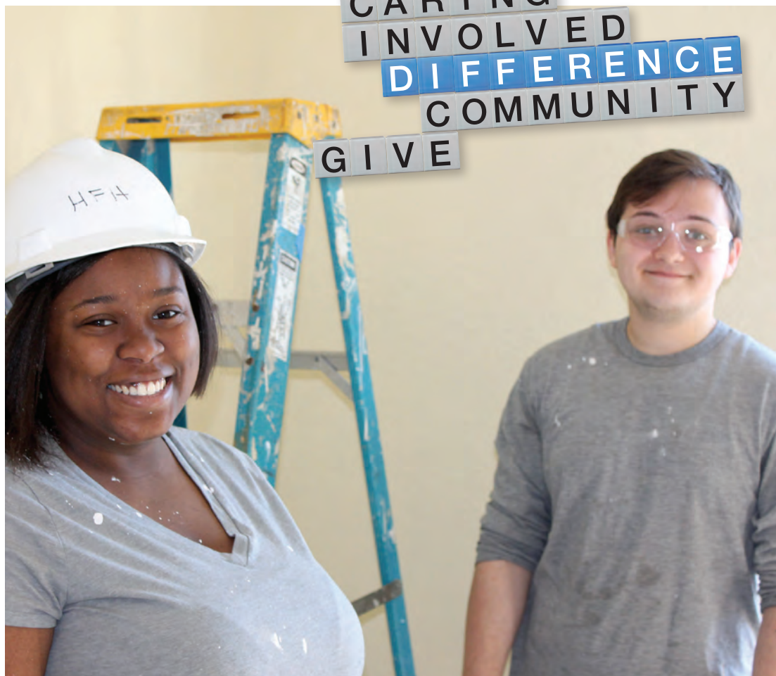
Berea College students Jade Garner '20 and Lee Myers '20 paint the interior of a home built by Habitat for Humanity.
