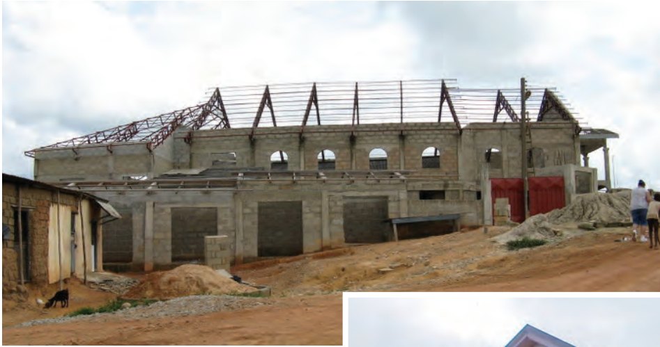
LEFT: In the Ghanaian village of Komfueku, the community was working to expand the St. John Church and Community Center when they ran out of money to complete the roof. Construction had halted when Dr. Valeria Watkins visited, and she pledged to raise the $25,000 necessary to complete the roof.
