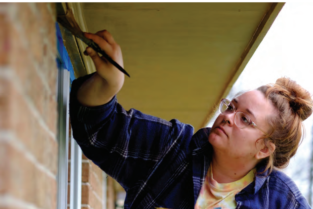
Lara Armstrong '18 paints the gold trim on an outside window. Lara and other members of the Spiritual Seekers group worked on this home with the St. Bernard Project during spring break.
