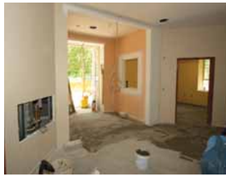
Upon completion the main lobby will provide a spacious entryway.
