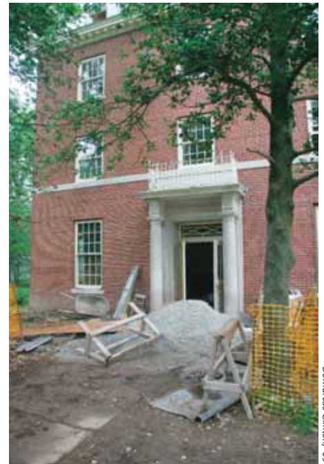
New energy efficient windows were installed this summer.
