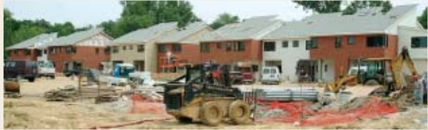
Construction on the Ecovillage has progressed rapidly this summer, with all apartments ready for occupancy this fall. Student families began moving in at the end of August.
