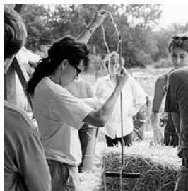
(Left) Buddy Williams, architect with Van der Ryn architects and a straw bale building expert, demonstrates how to divide a straw bale to fit the dimensions of the shed. (Right) Participants use human energy to make plaster.
