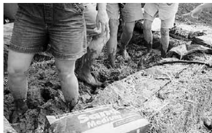
(Left) Buddy Williams, architect with Van der Ryn architects and a straw bale building expert, demonstrates how to divide a straw bale to fit the dimensions of the shed. (Right) Participants use human energy to make plaster.
