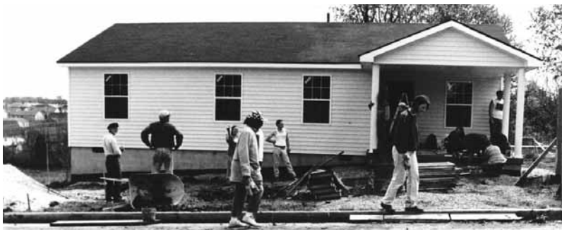
The house for the Lewis family was nearing completion in late April.
