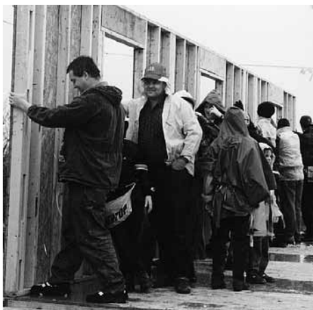
Students, faculty and staff help raise the first wall for the Joe Lewis home. The house on Mary Street was completed and dedicated in May.
