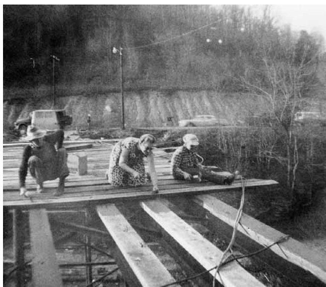
Irma Gall (center) and two others are shown repairing a bridge in 1966 for facilitating transportation to the Lend-A-Hand Center. The bridge, constructed in 1960, needs to be repaired every six-eight years.
